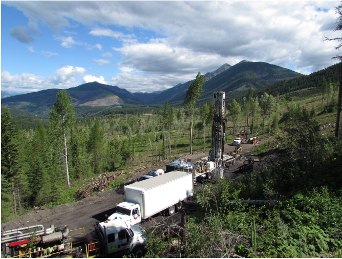
Fig. 17. Large diameter core hole drilling on the Loop Ridge property (CanAus Coal Ltd.), for coal quality testing. Looking north towards the Elkview mine.
