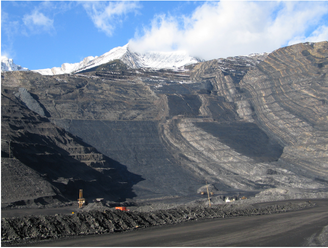
Fig. 12. Coal seams in the Alexander Creek syncline at the Line Creek mine. Photo courtesy of Teck Coal Ltd.
