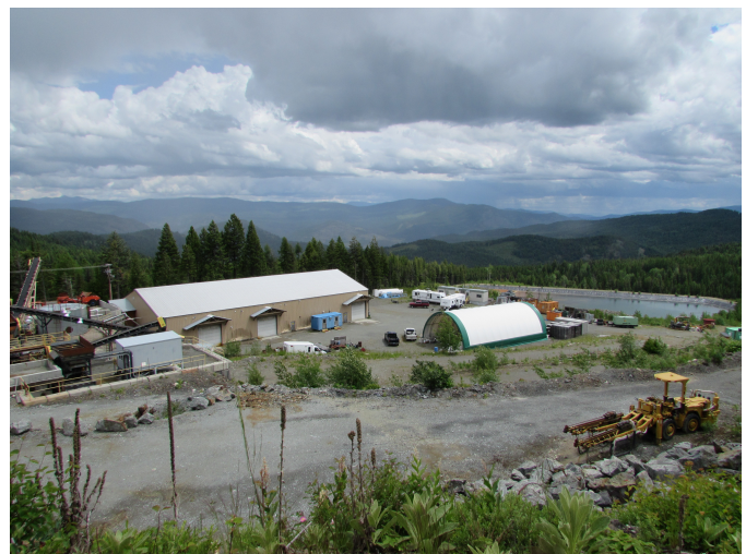
Fig. 19. The 200 ton-per-day Lexington mill (gravity-flotation) and tailings facility. Golden Dawn Minerals Inc. has entered into a purchase agreement with Huakan International Mining Inc. to acquire both the Lexington mine and mill, as well as the nearby Golden Crown mine. Both mines are underground Cu-Au mines.
