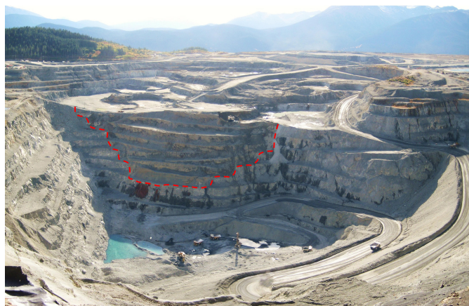
Fig. 5. Looking west-southwest over the Huckleberry Main Zone Extension pit. Year four of the Main Zone Optimization plan continued to remove formerly deposited tailings to recover ore below and around the former Main Zone Pit (former Main zone pit outline highlighted by dotted red line). Photo courtesy of Justin Schroff, Huckleberry Mine geologist.
