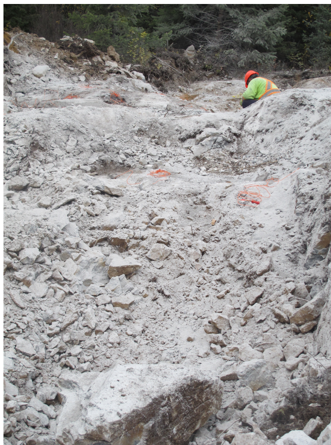
Fig. 12. Loading blast-holes at Giscome.
